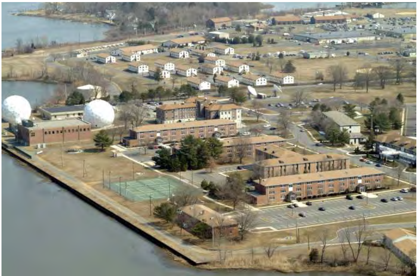
World War II barracks and training facilities in the background with visiting quarters in the foreground.
